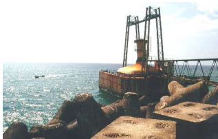
OWC installed in 1990 at Trivandrum, India.
