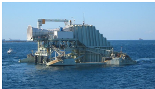
OWC installed in Australia, about 2005.
